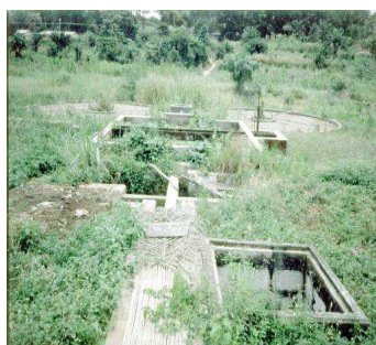
▶ figure 1: defunct sewage treatment system, Kumasi, Ghana from the 1970s
